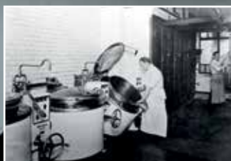
First generation of tilting boiling pans 1934
